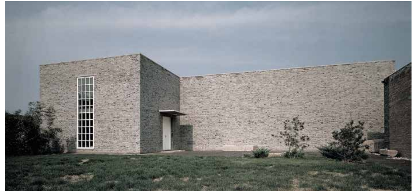
Studio House, Caochangdi, Beijing, 1999.
